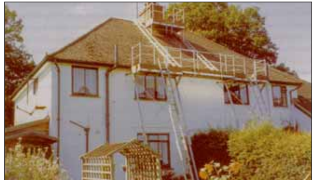
Figure 3 Proprietary access system for roof work
